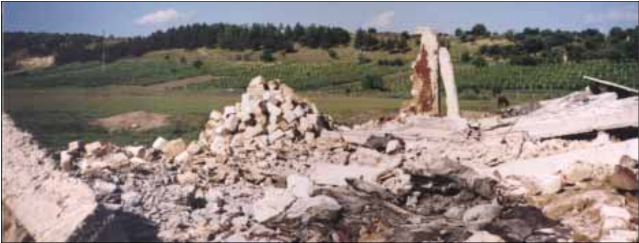
▲ Destroyed storehouse, Lapusna, Hincesti rayon
