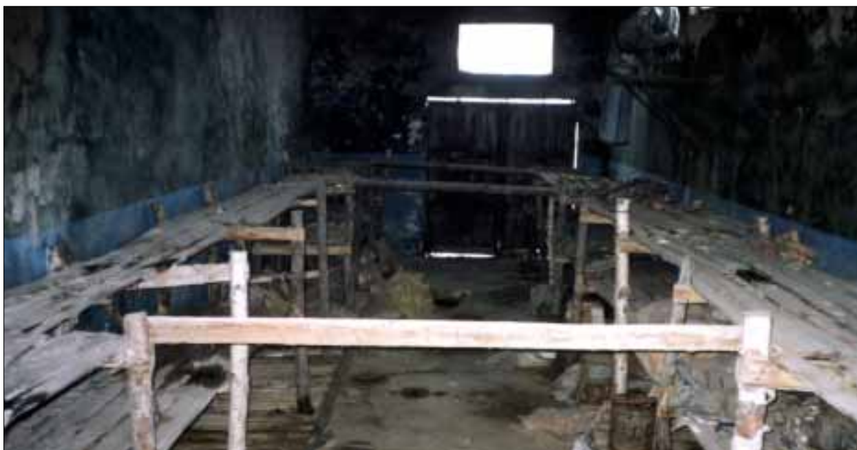
▲ Clean-up of warehouses is planned.
