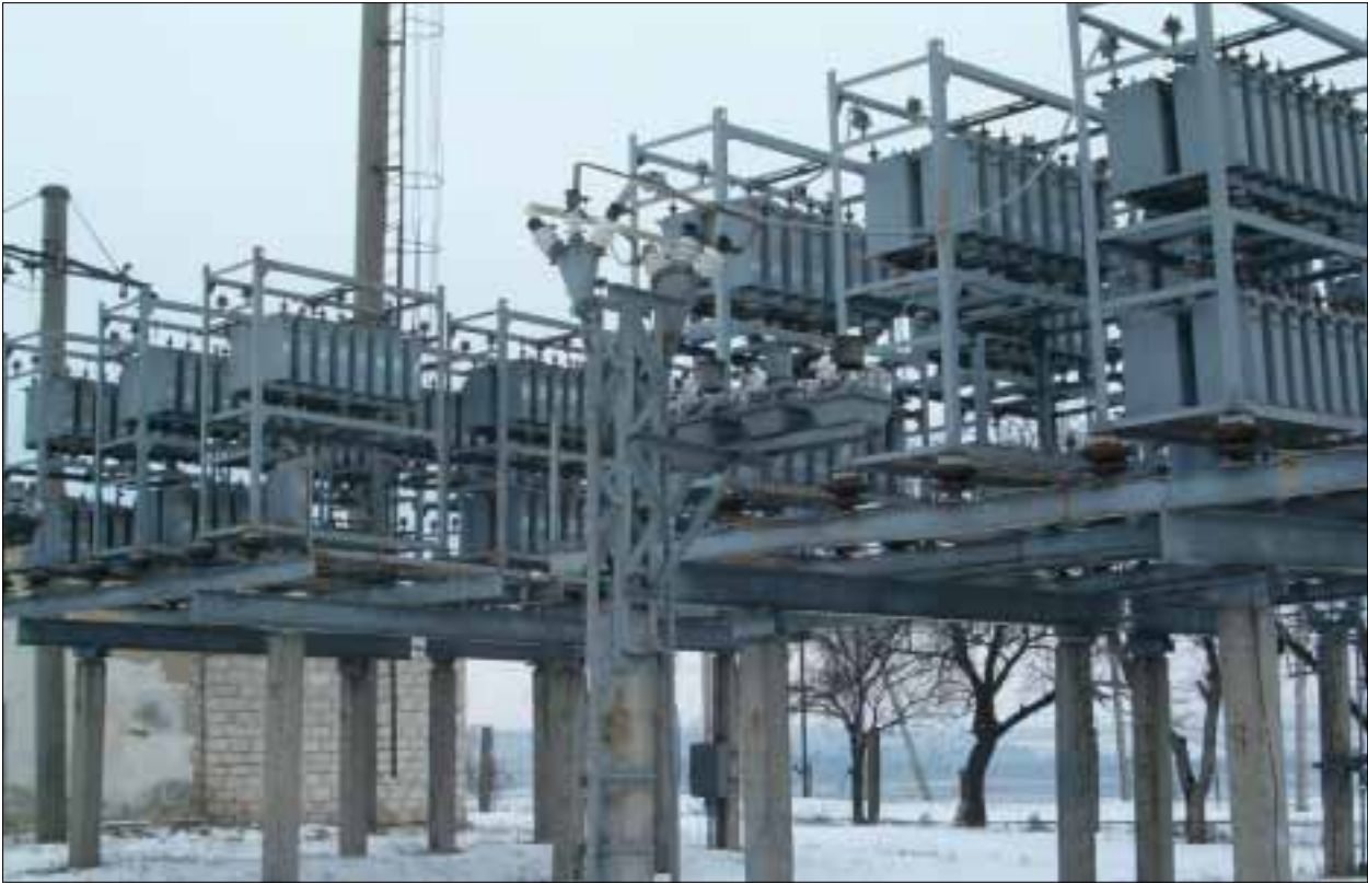
▲ General view of a block of capacitors, Orhei
